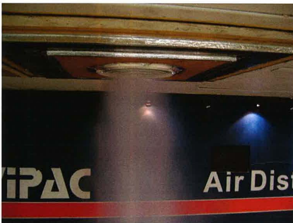
Figure 10: Jet Ceiling Diffuser (Neck: Ø300mm).
